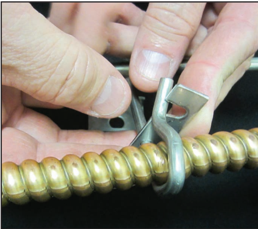
Horizontal supports for VITALink® Armored cable.
