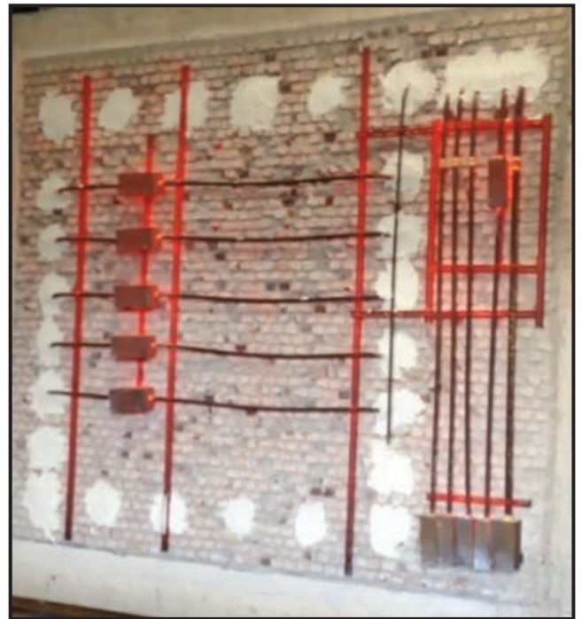
After wall is removed from furnace
