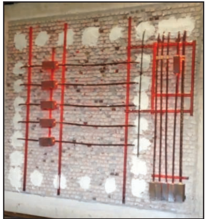
After wall is removed from furnace
