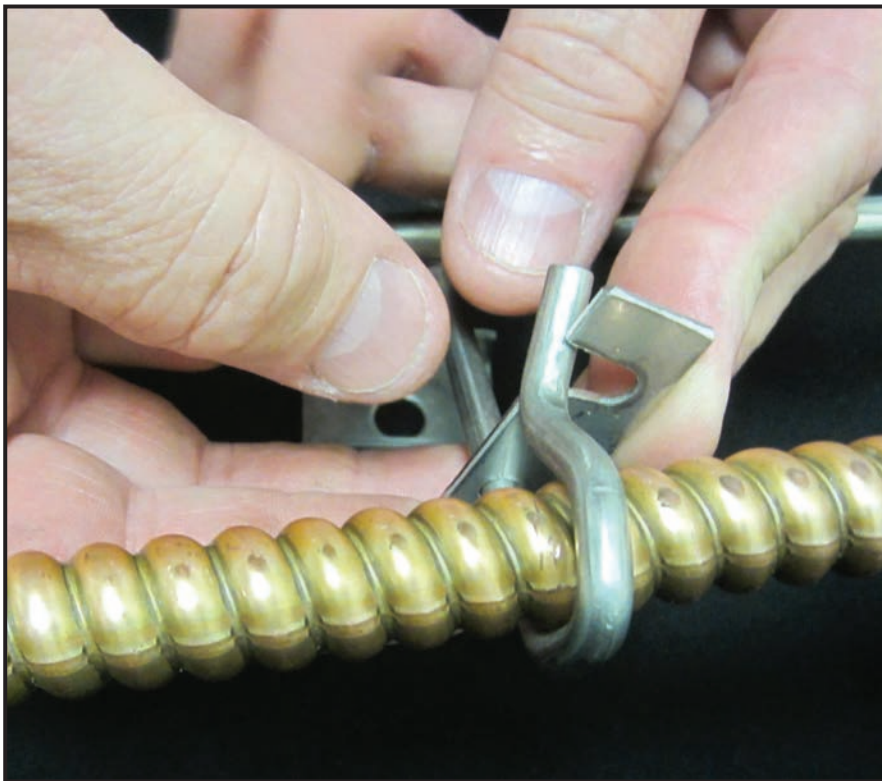
Horizontal supports for VITALink® Armored cable.
